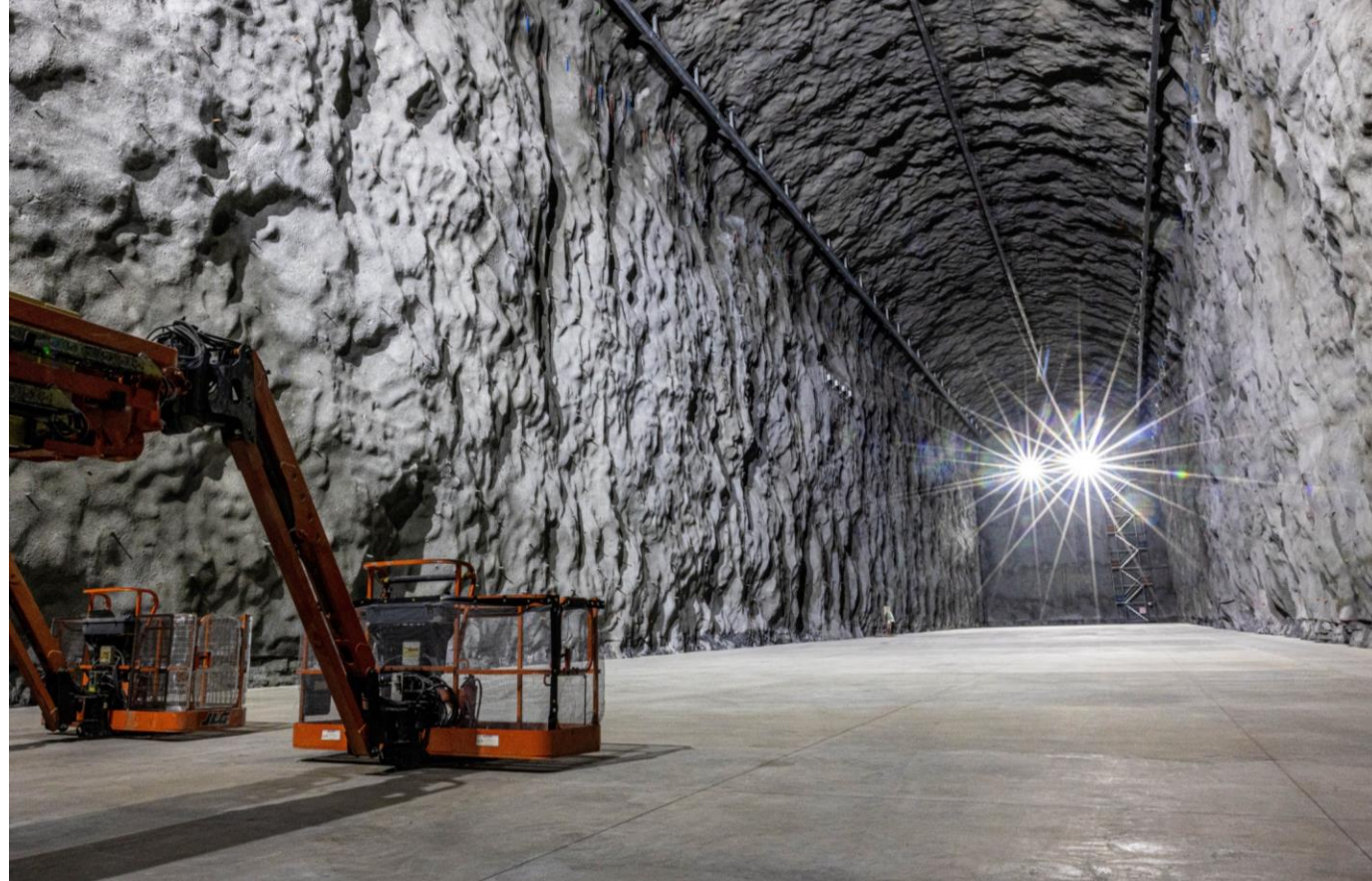
Far Detector Cavern – excavation and concrete complete!
