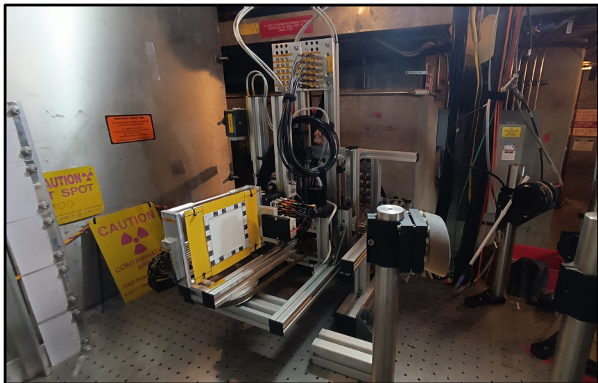
Installation at the FACET-II dump table
