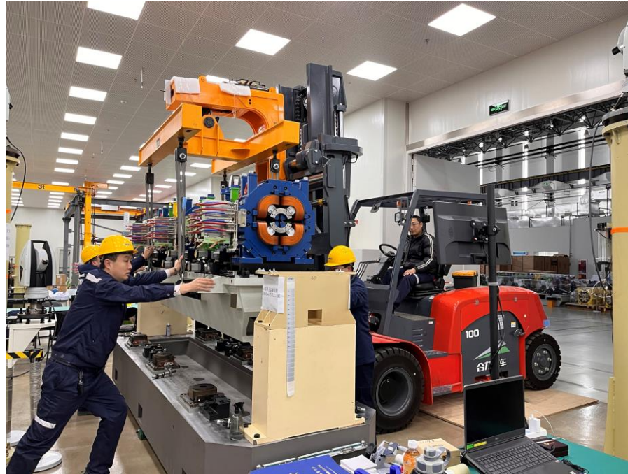
replacing the girder
