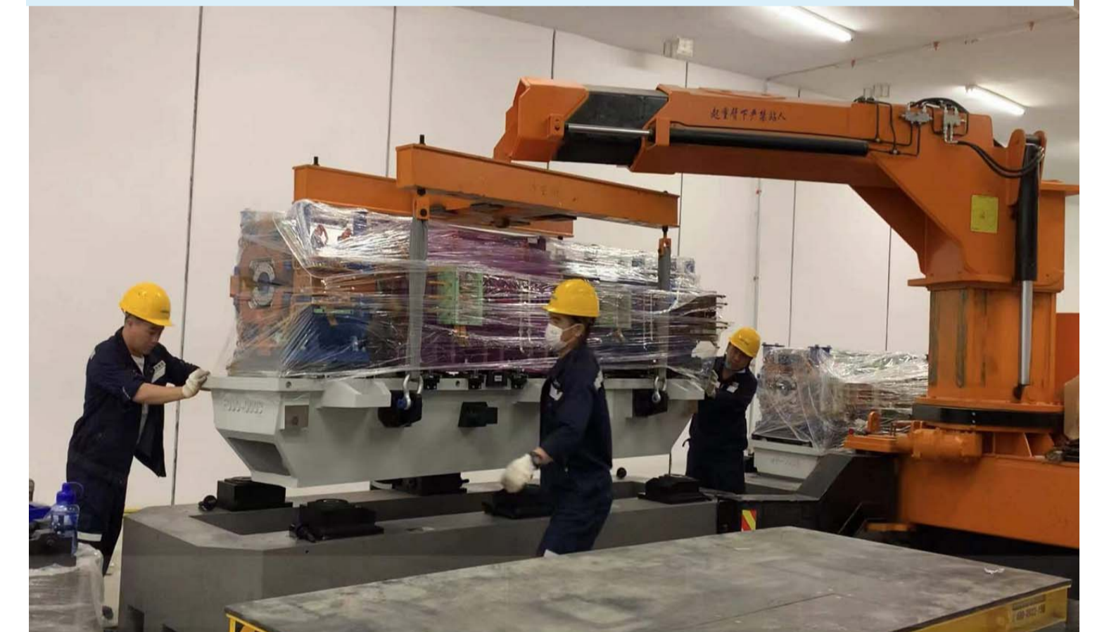
Installation of the pre-alignment units
