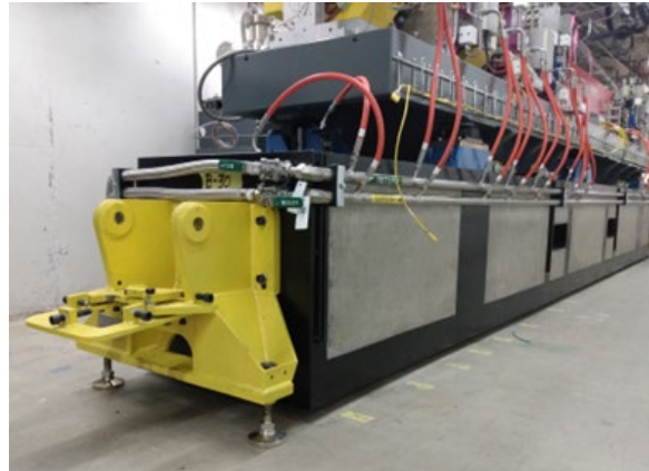
Figure 6: Plinth end rigger support for module for grouting.
