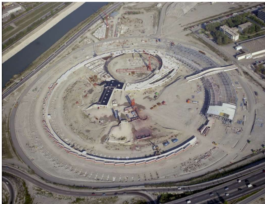
Figure 2 The construction of the ESRF in 1990.
