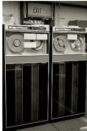
Reel to reel tape drives. Reels mounted by hands! 140 Mbytes/Reel
