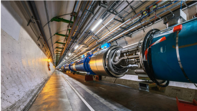
LHC Dipole in Tunnel
