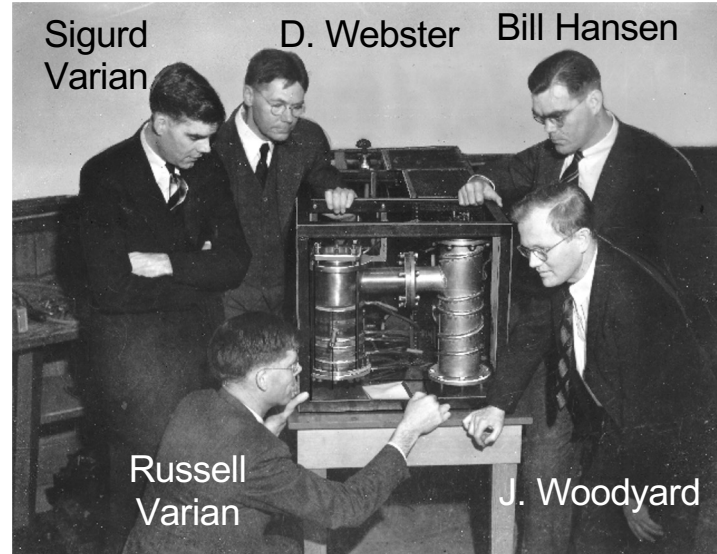
250 MHz klystron used for the U.S. Army blind landing system before World War II, Stanford University, 1939.
