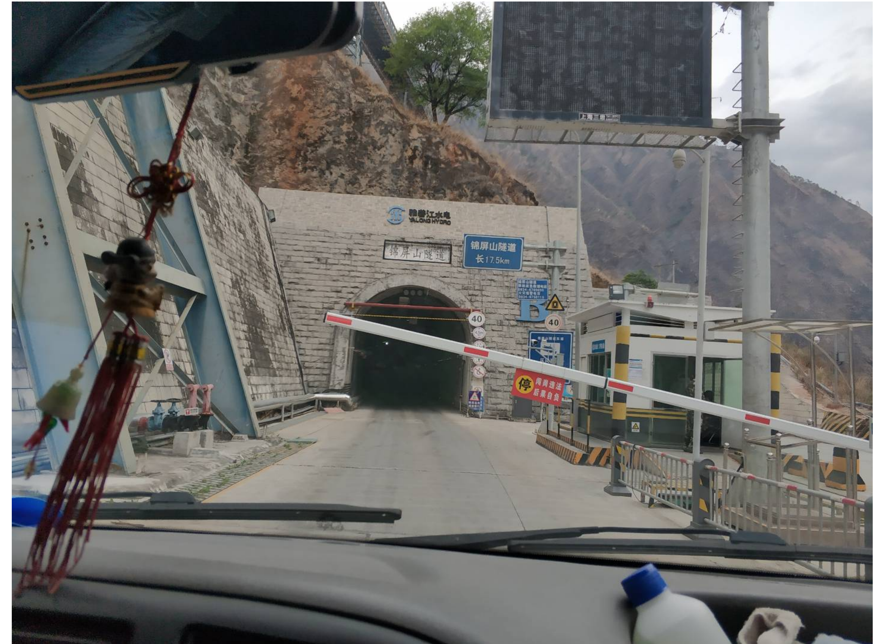
drive into tunnel
