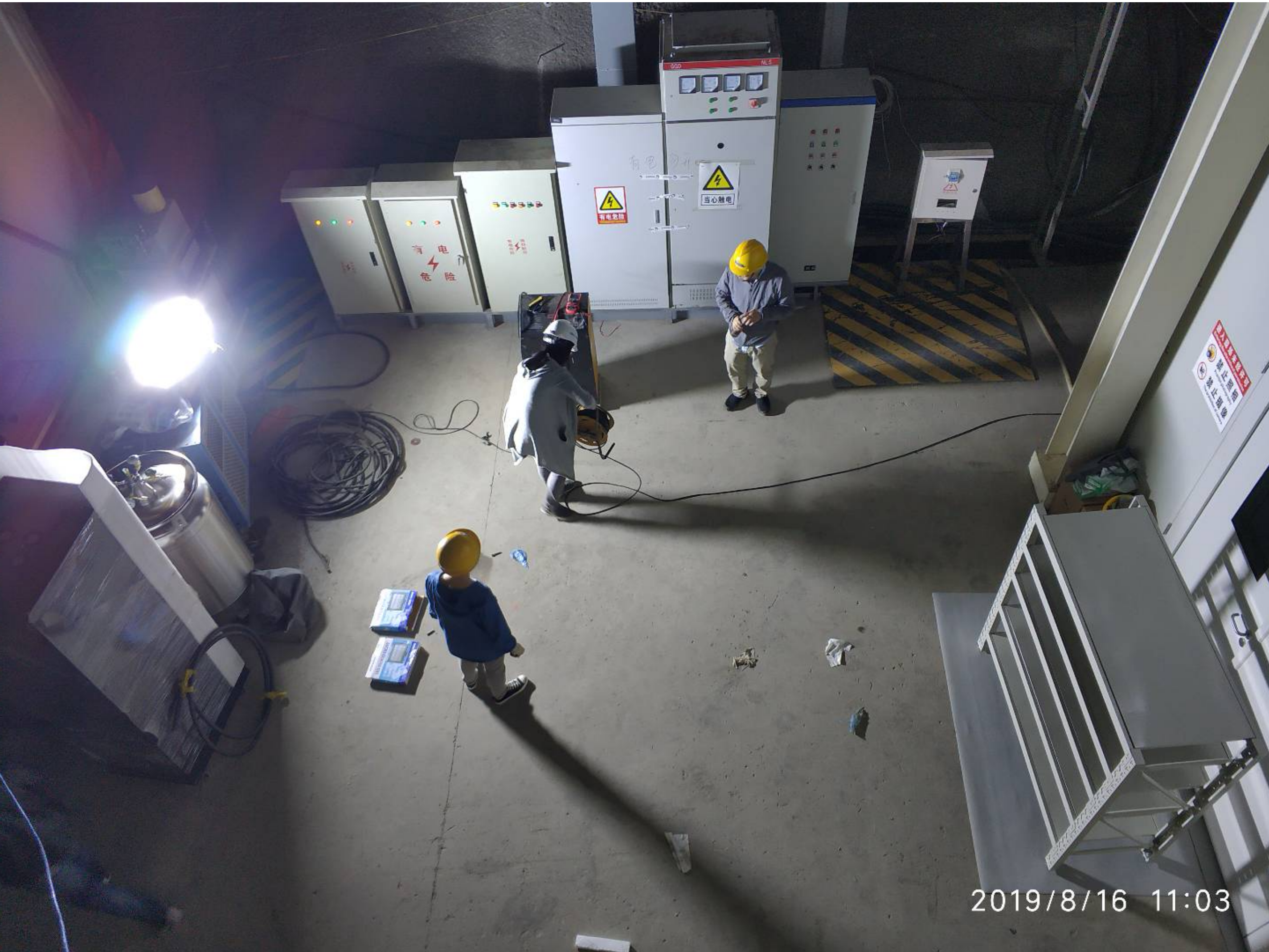
fix electric infrastructure by ourselves
