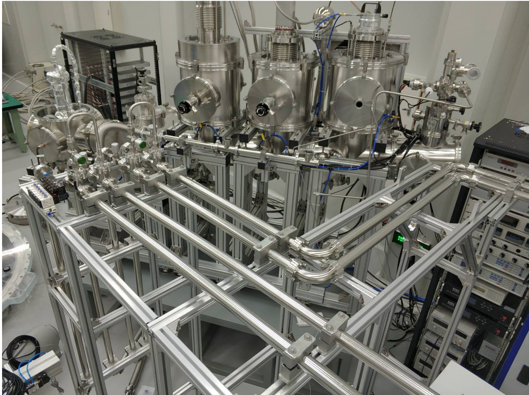
cooling bus and circulation
