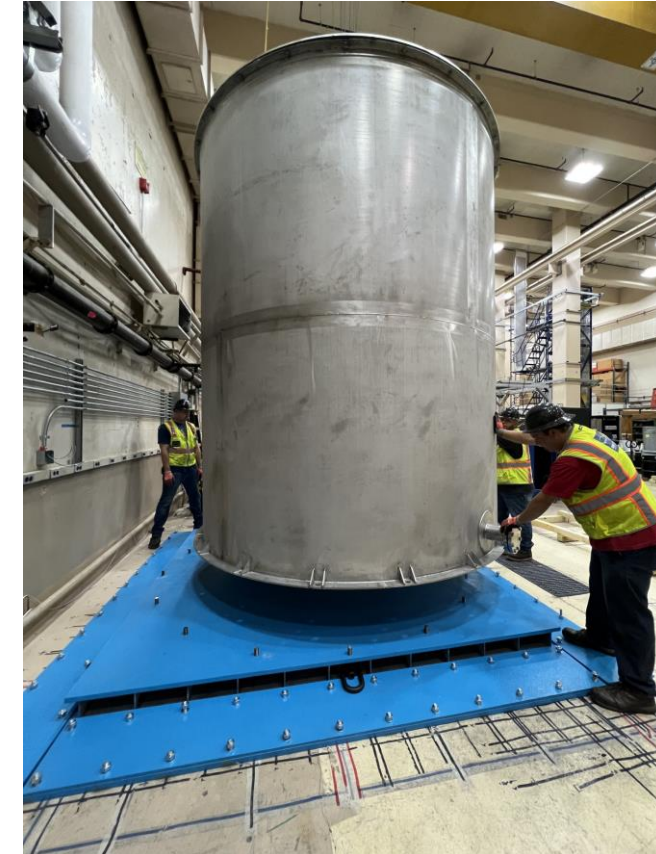
Outer vessel (OV) lowered onto seismic anchorage base plates
