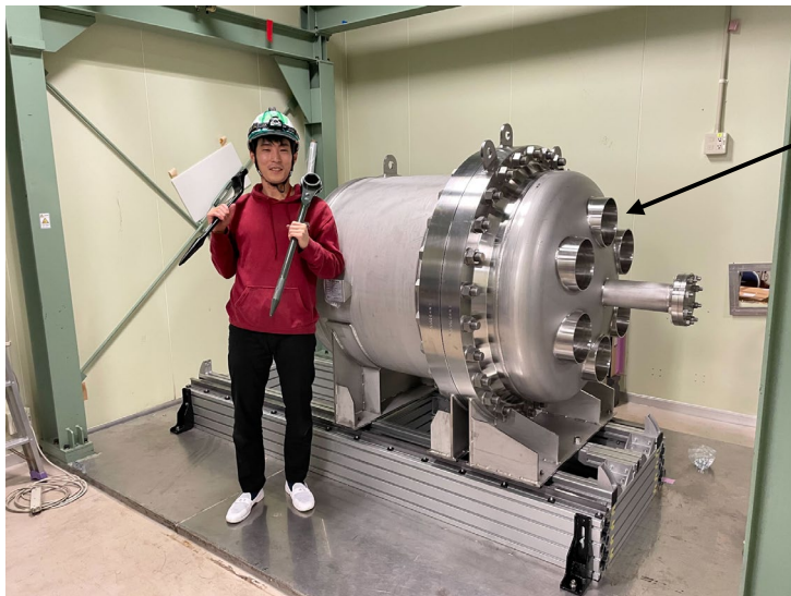
installation of pressure vessel
