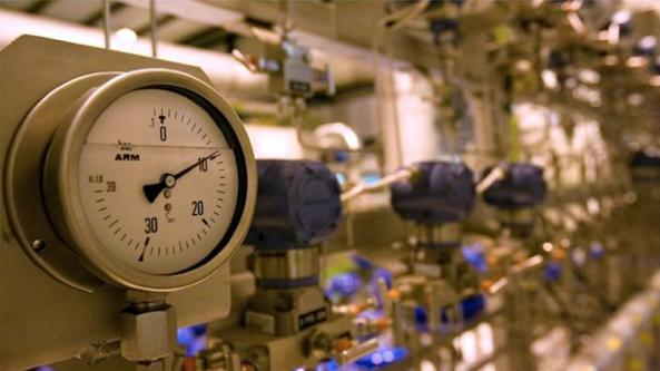
A pressure gauge at the Large Hadron Collider's cryogenics, which take up more than half of the accelerator's electricity consumption. Credit: Adam Hart-Davis/SPL
