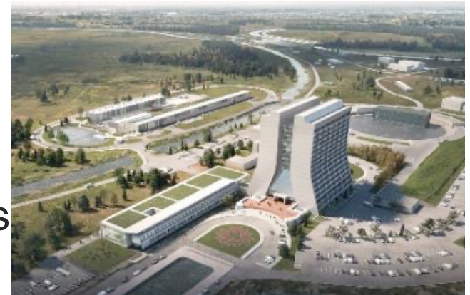
Fermilab Accelerator Complex with the new PIP-II Linac (under construction)
