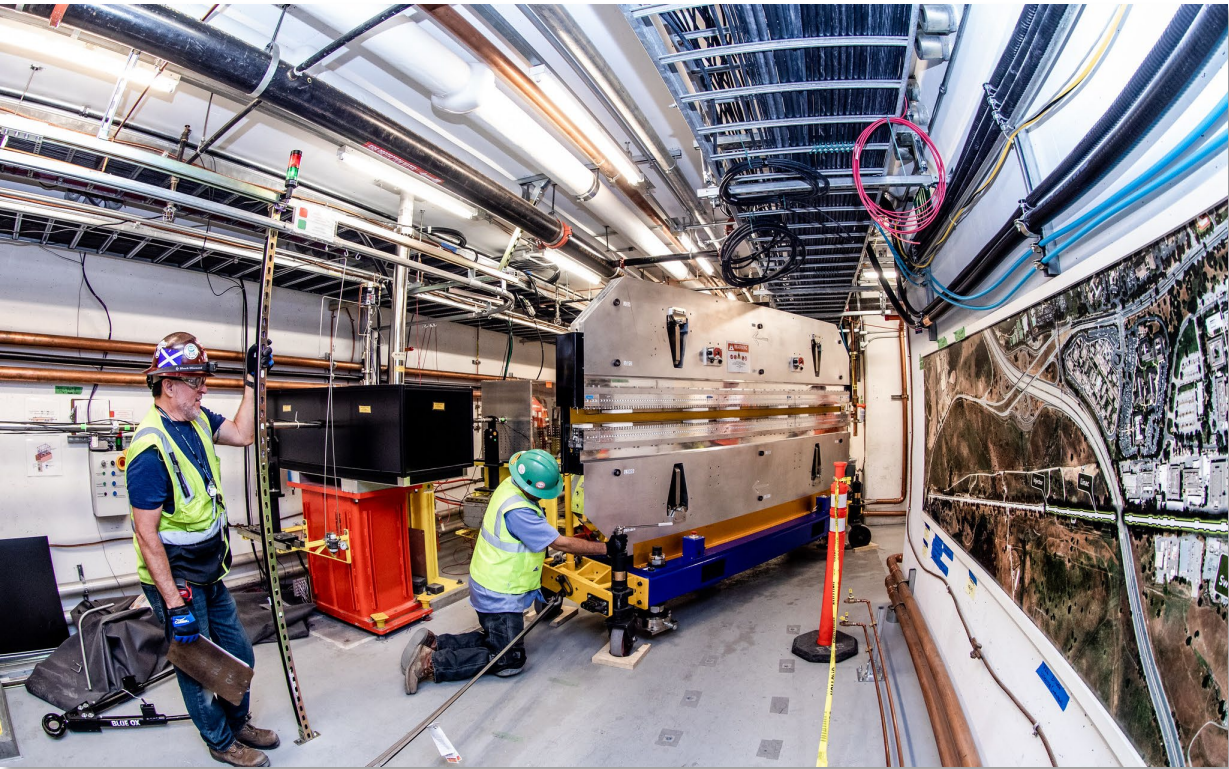
Vertical Variable Gap SXR Undulator
