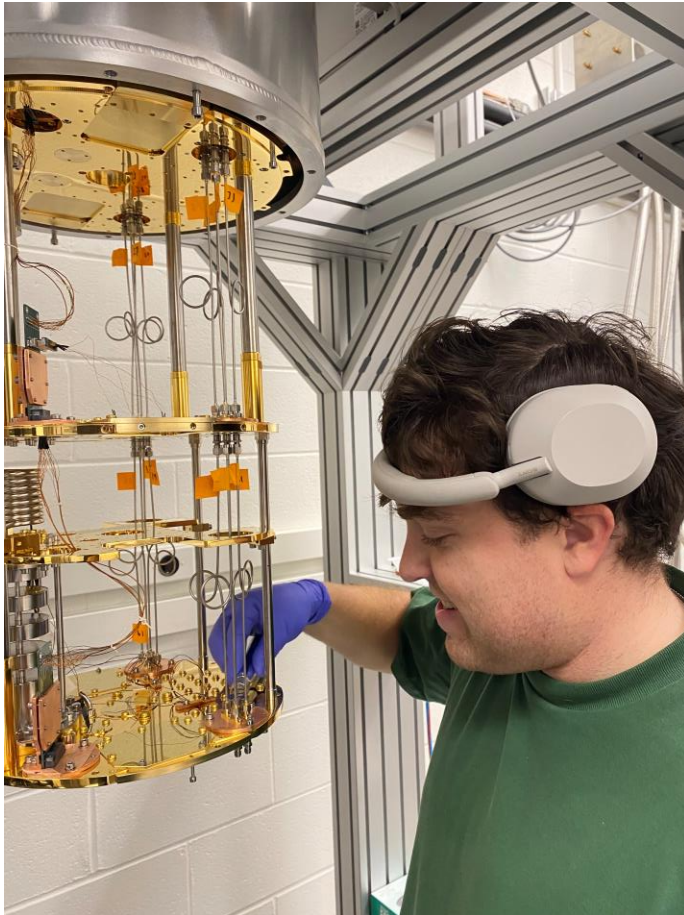
Joe installing coax in DR
