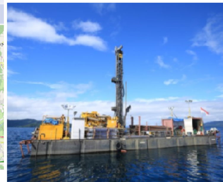
Drilling works on the lake
